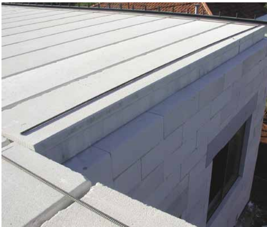
Image 7.3.2: Installed Floor Panels
