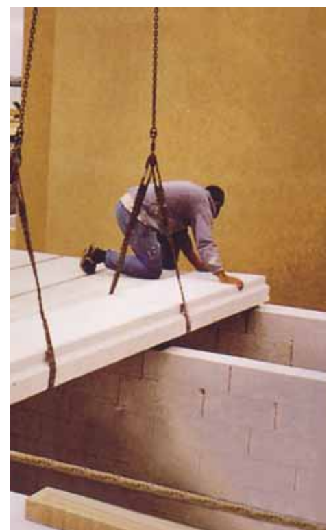
Image 7.3.3: Installing Floor Panels
